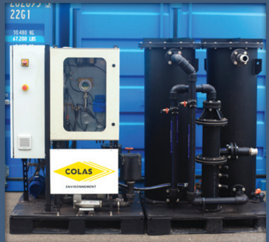
Figure 2 - Skid de Venting
