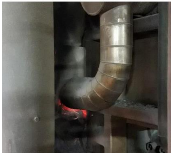
Figure 5 : Lateral crack in the furnace
