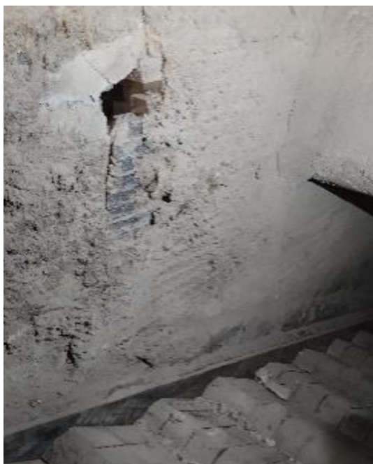
Figure 13 : The projection of a fragment of a nitrous oxide canister into the furnace
