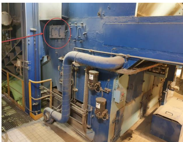
Figure 10 : Hatch blown off by the blast of the explosion
